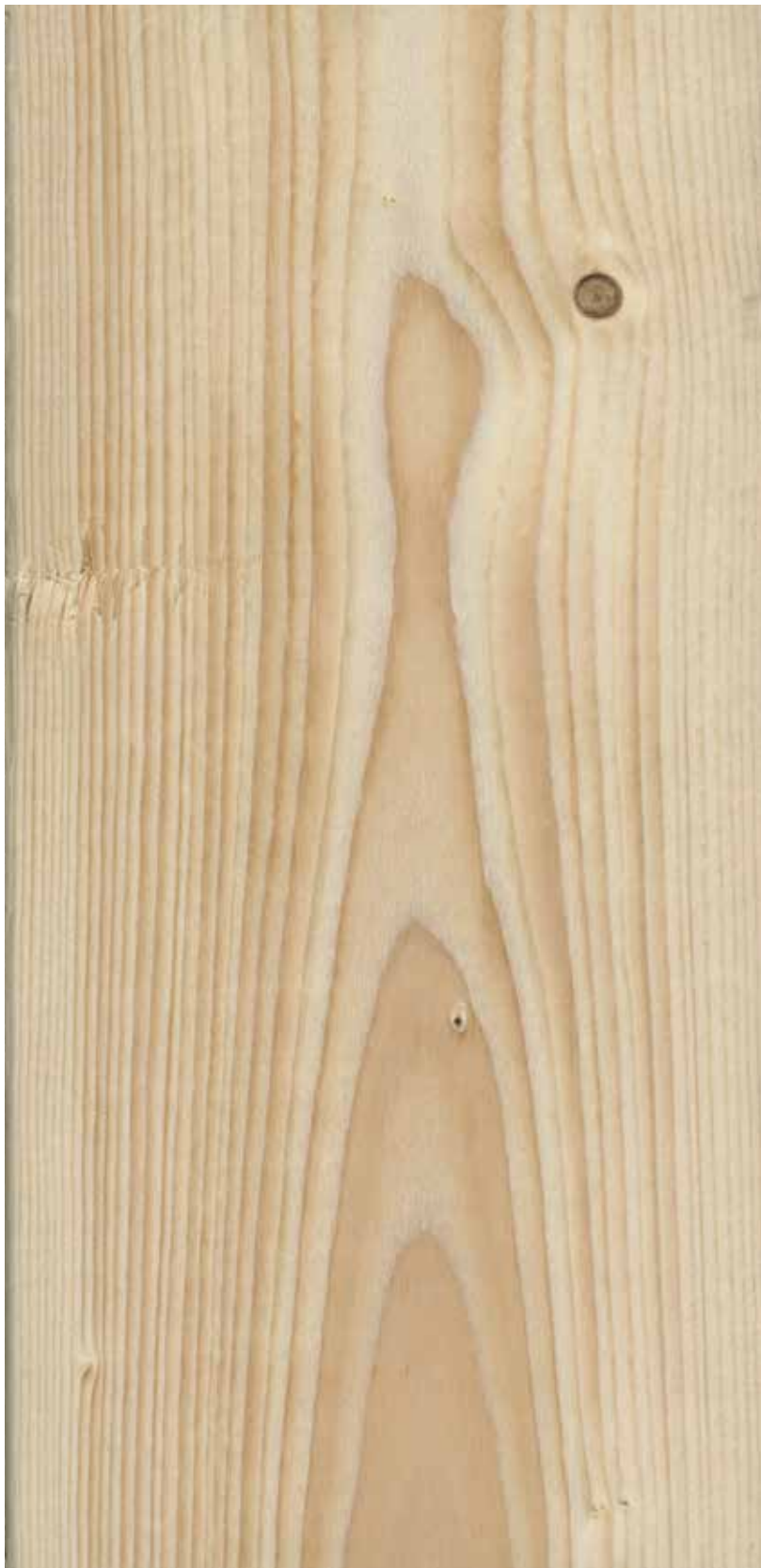
Figur 66. Forholdvis stor skade, planken vrakes.
