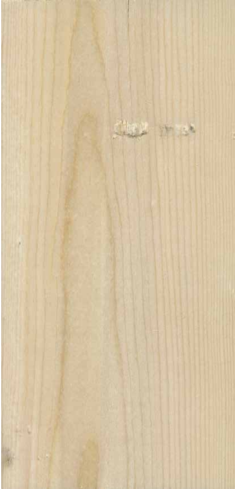
Figur 67. Forholdvis stor skade, planken vrakes.
