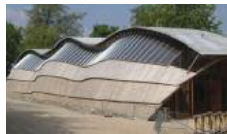
The Downland Gridshell. Foto: Green Oak Carpentry
