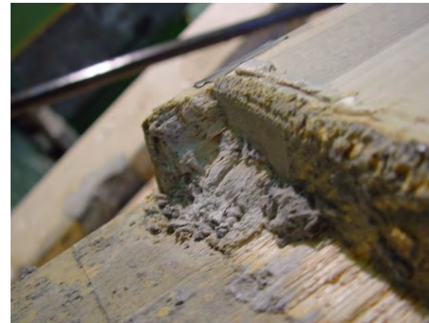
Crushing of timber
