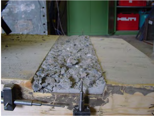
Shearing of concrete
